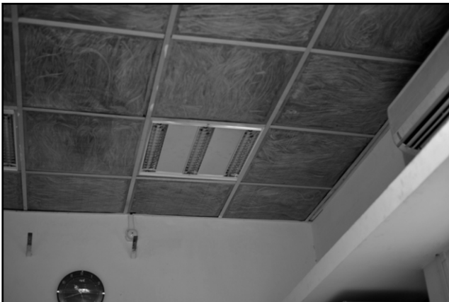
Figure 4: Jute based fibers used as ceiling tiles
