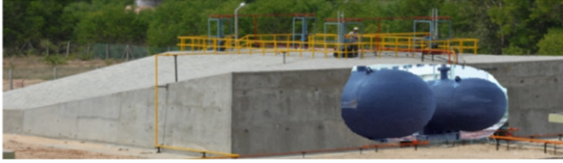
Fig. 9 - LPG storage system
