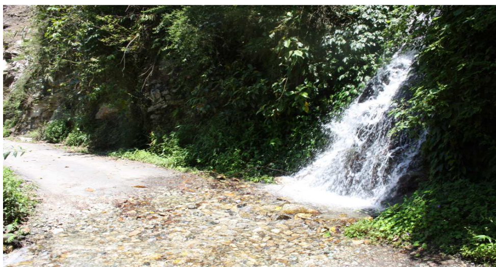
Roing- Etalin Road "Water Falls- Directly discharging on the Road having No Culverts
