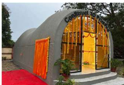
Fig. 5 - 3D Print Pod using Ultra-High Performance concrete with fibres
