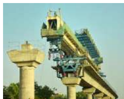
Precast Elements Using Heavy Machinery
