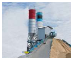
Modern Batching Plant
